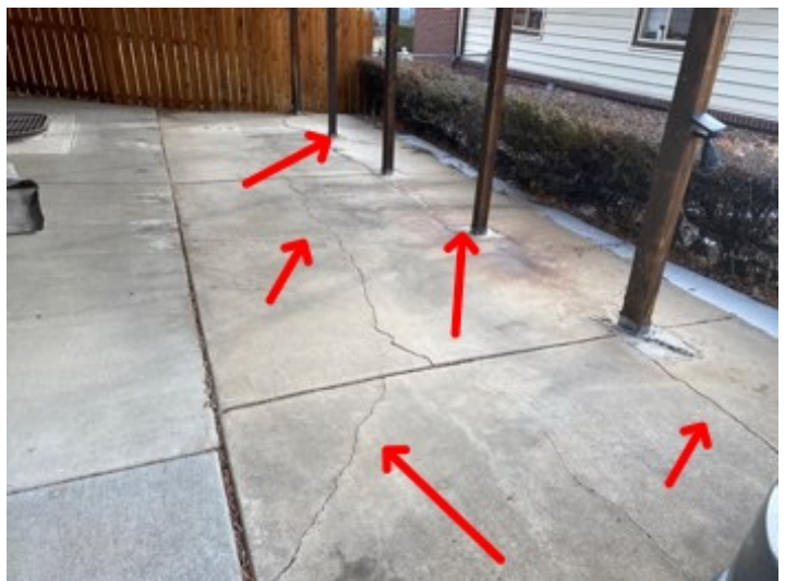
Cracking noted recommend Caulking and monitoring
