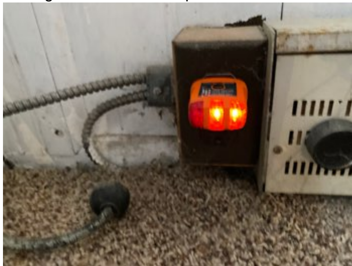
Un-grounded not GFCI protected outlet noted
