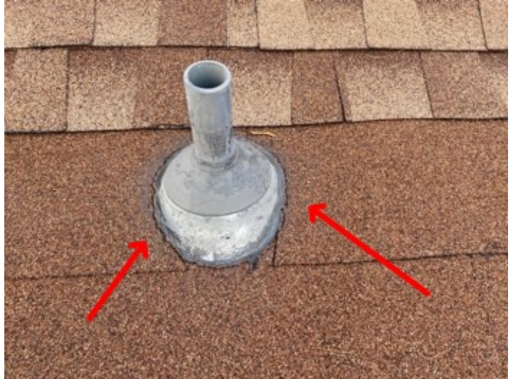
Caulking recommended to locations inch and a half vent pipe
