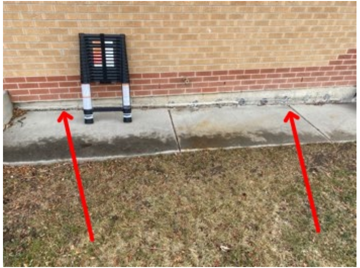
Settlement noted recommend re-caulking to prevent water infiltration
