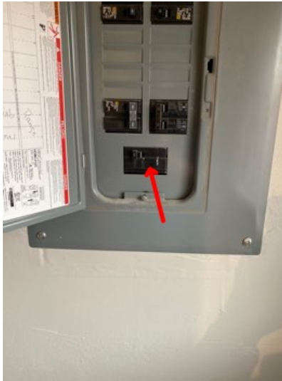
Main Electrical Shutoff
