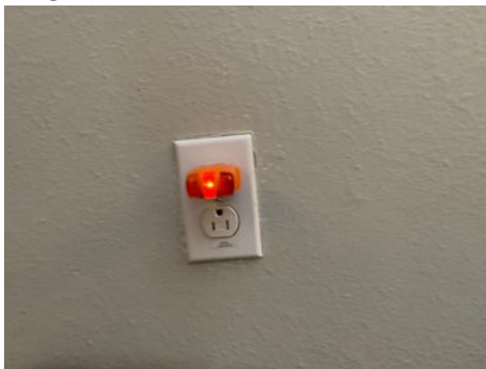
Un-grounded not GFCI protected outlet noted
