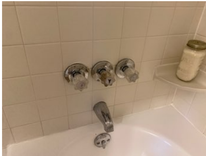
Shower plumbing is loose is wall
