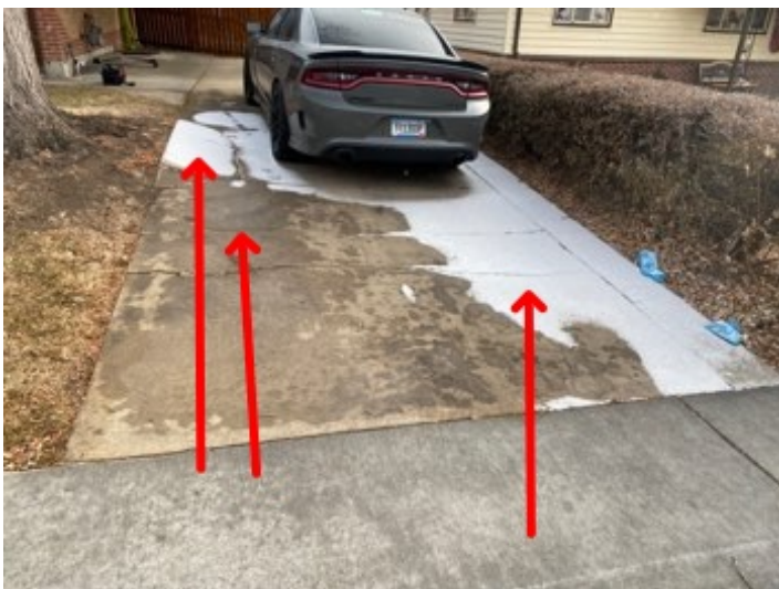
Cracking and heaving noted
