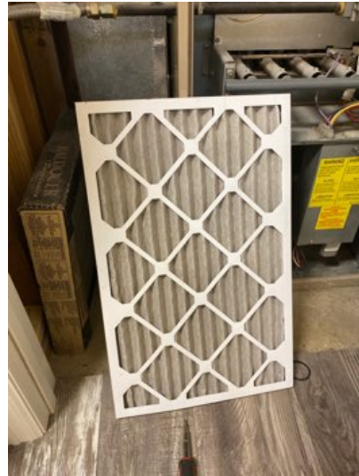
Recommend filter replacement every three months at least. 16x25x1
