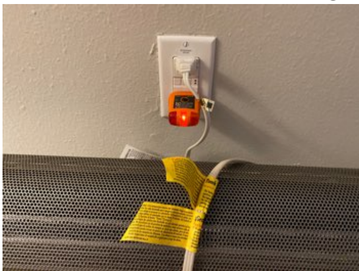
Example of un-grounded GFCI protected outlet
