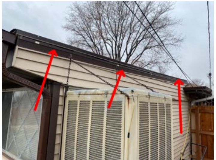
Missing flashing noted water can enter wall covering behind siding recommend repairs by qualified contractor
