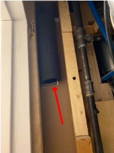
Combustion air covered by pipe insulation recommend removing insulation
