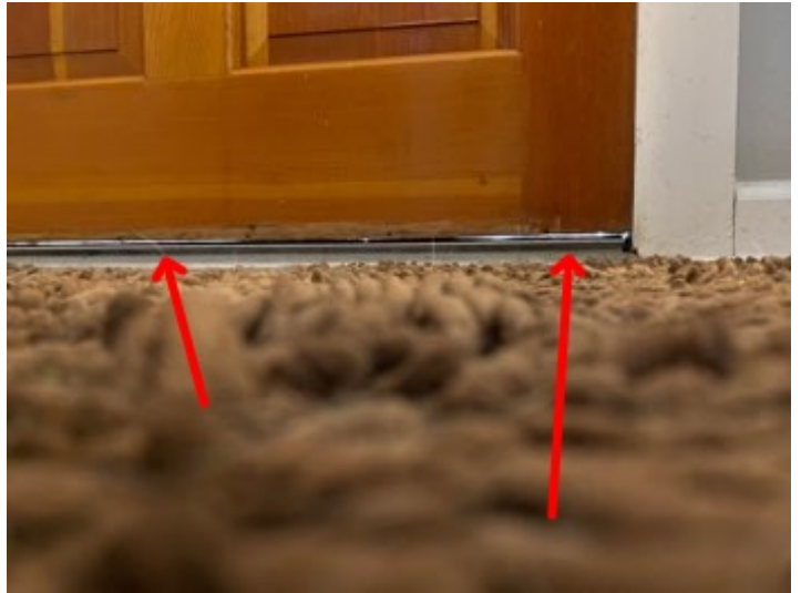
Daylight visible at door bottom, Recommend repairs by qualified contractor
