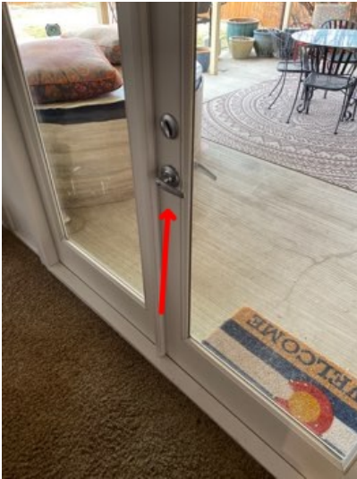
Door did not latch, recommend repairs by a qualified contractor
